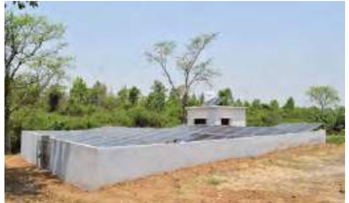
Solar Irrigation Project
